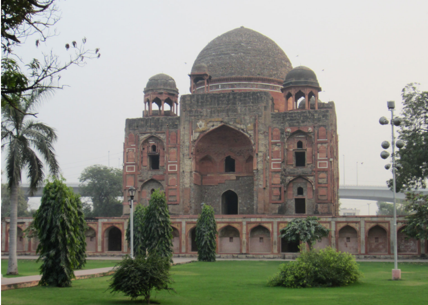
FIGURE 10.4 The mausoleum of 'Abd al-Rahim khān-i khānān (1556-1627) in Delhi. Photograph by Richard McClary
